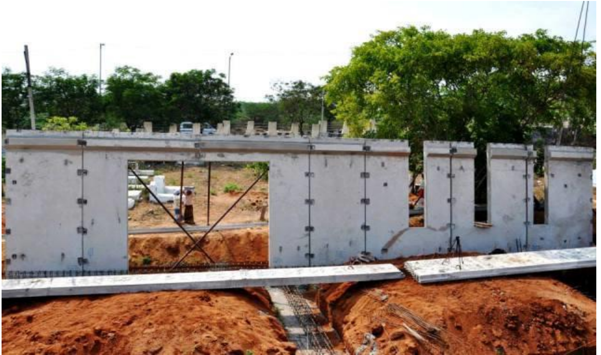
Erection of Engraved panels
