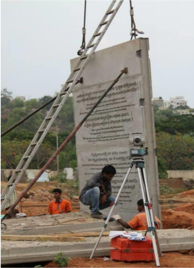
Erection of Engraved panels
