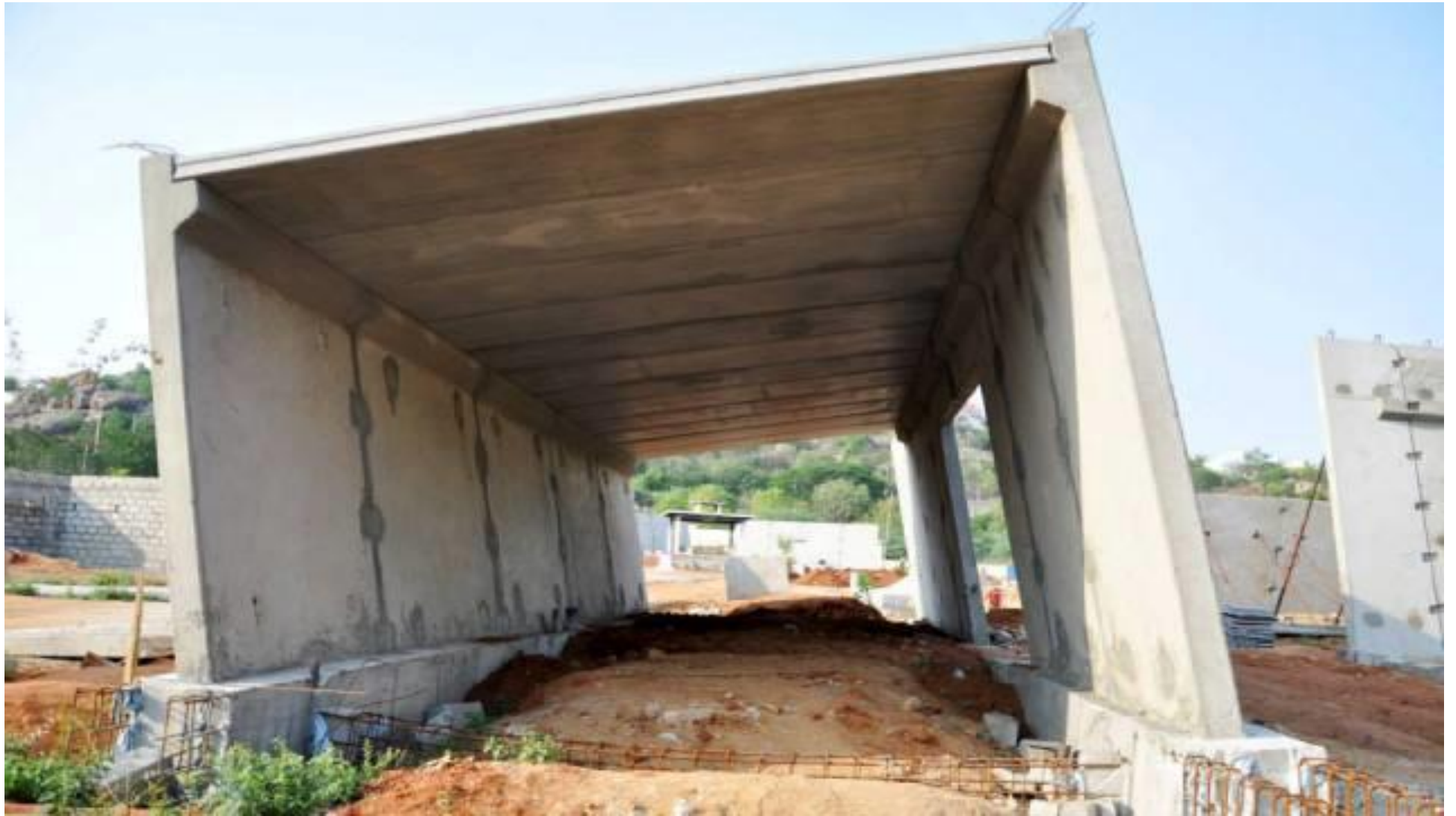
Erection works in progress
