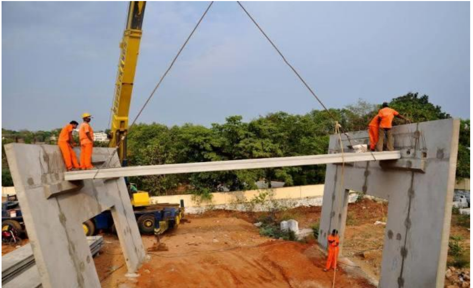
Erection of Hollow Core Roof Slabs
