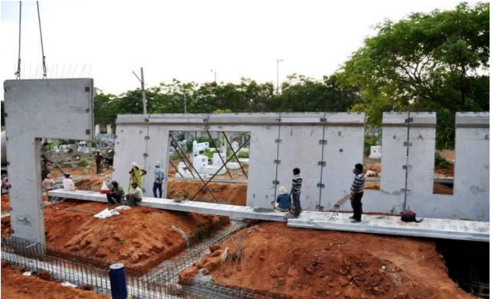
Erection of Engraved panels
