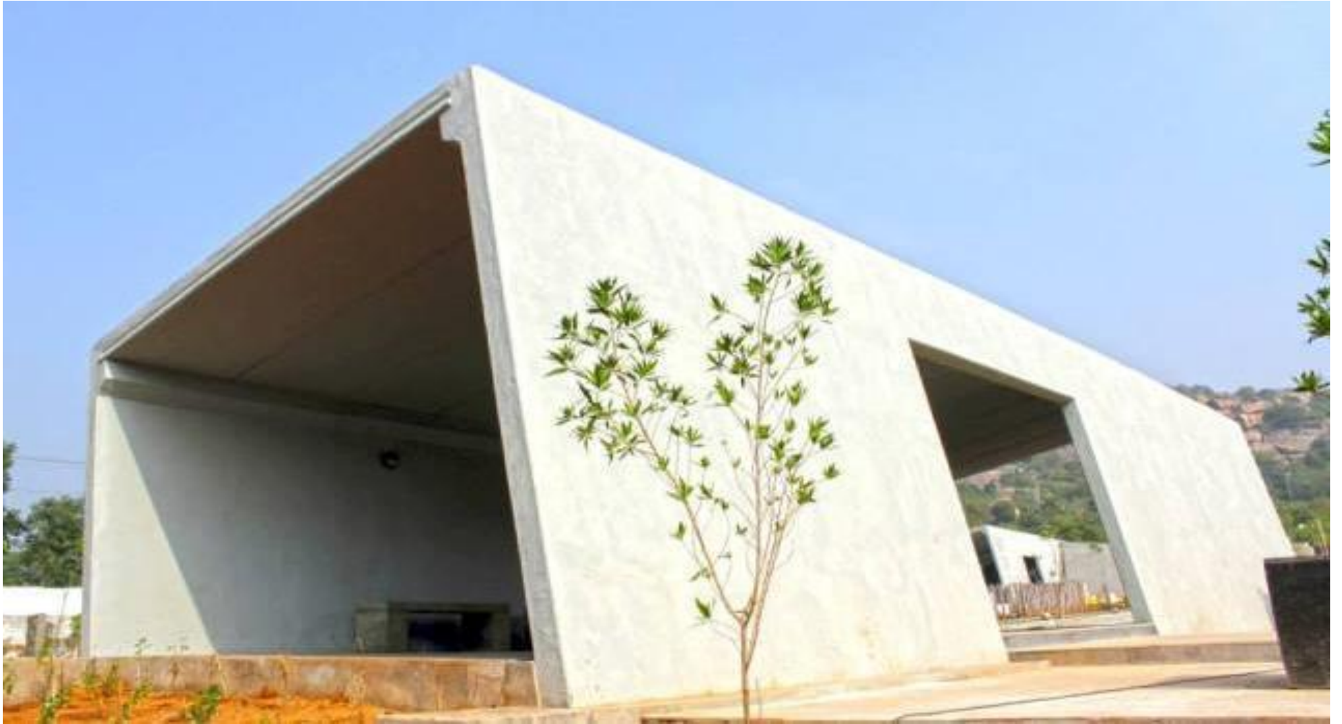
Completed Crematorium Shed - 2
