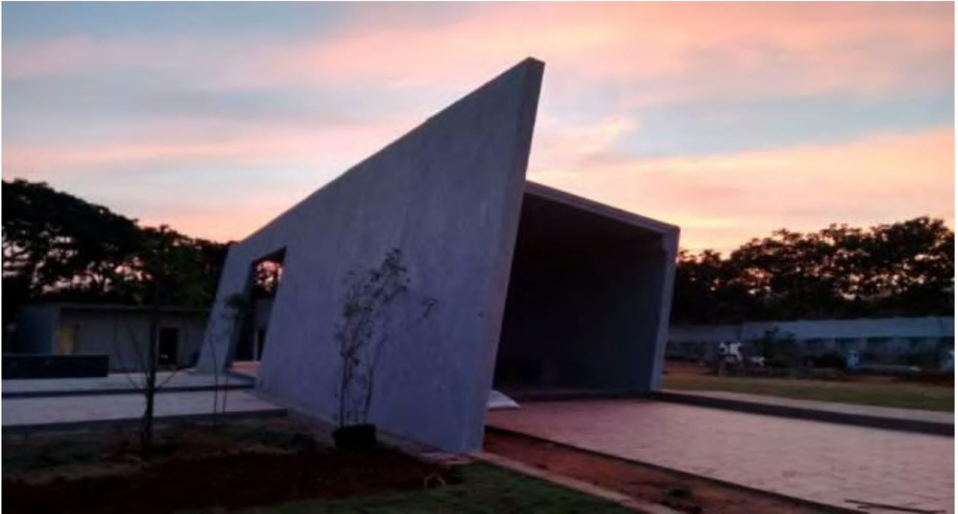
Completed Crematorium Shed -3
