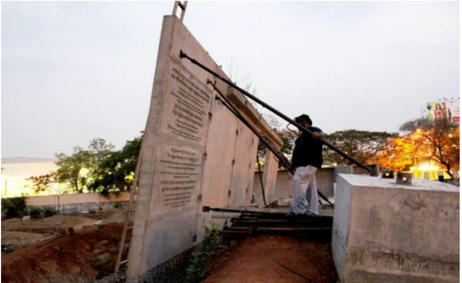
Erection of Engraved panels
