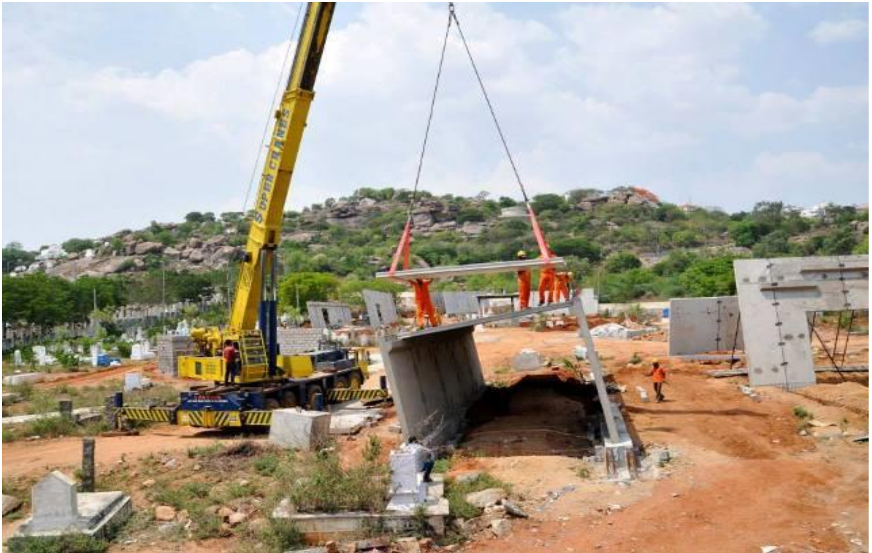
Erection of Hollow Core Roof Slabs
