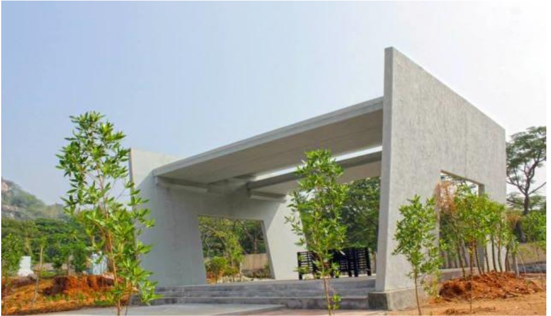
Completed Crematorium Shed - 1
