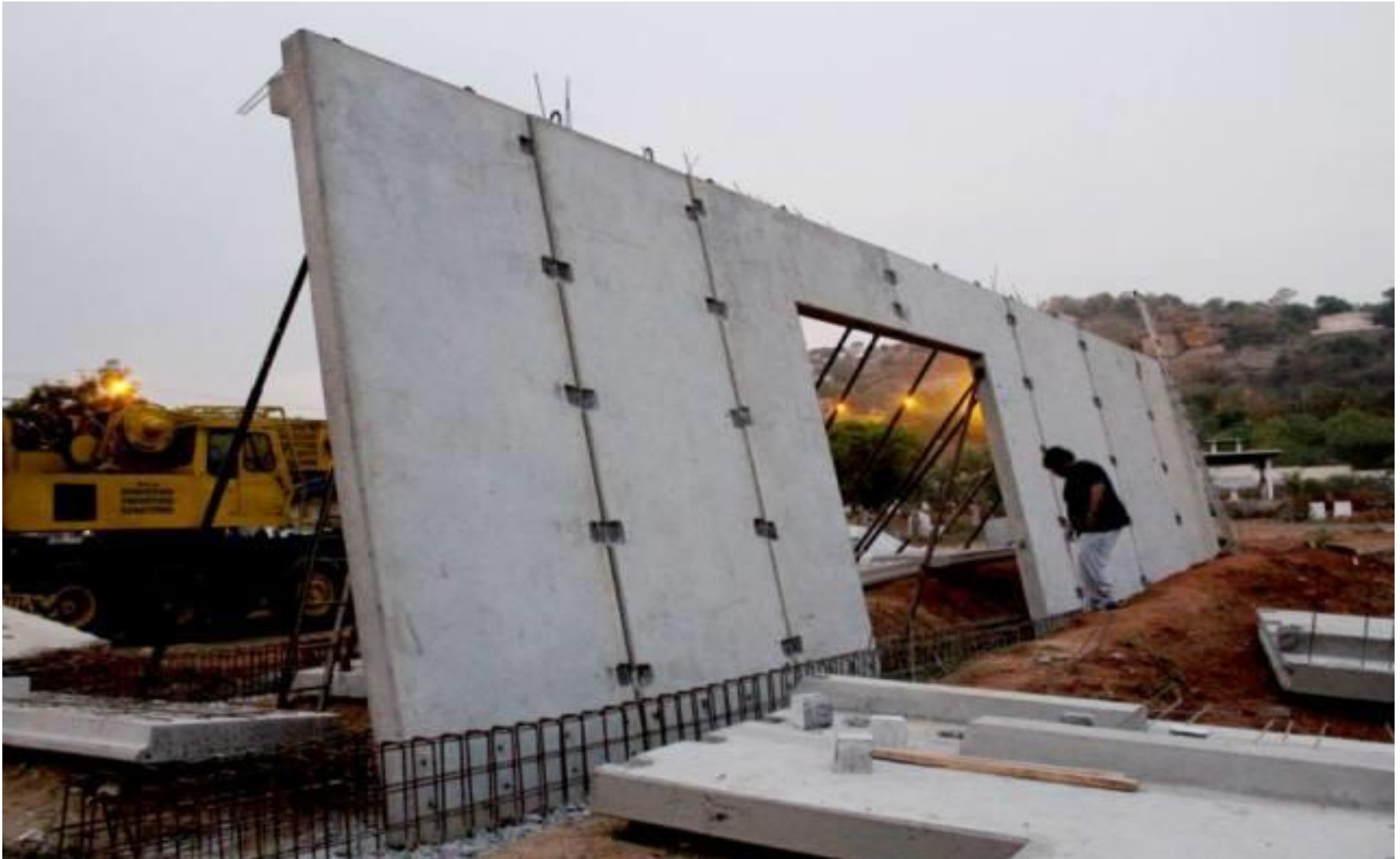
Erection of Engraved panels
