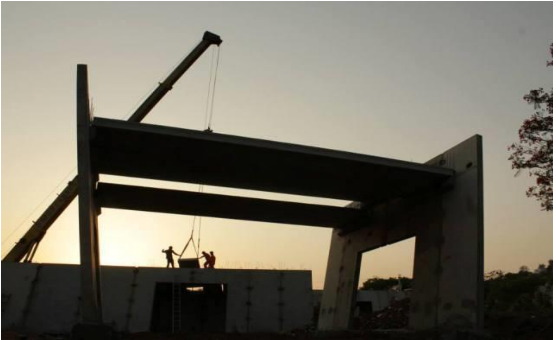
Erection of Hollow Core Roof Slabs
