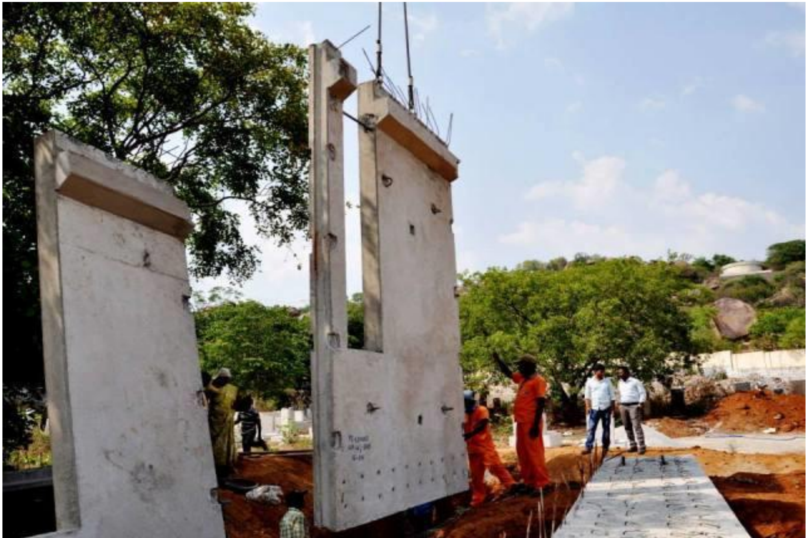
Erection of Engraved panels
