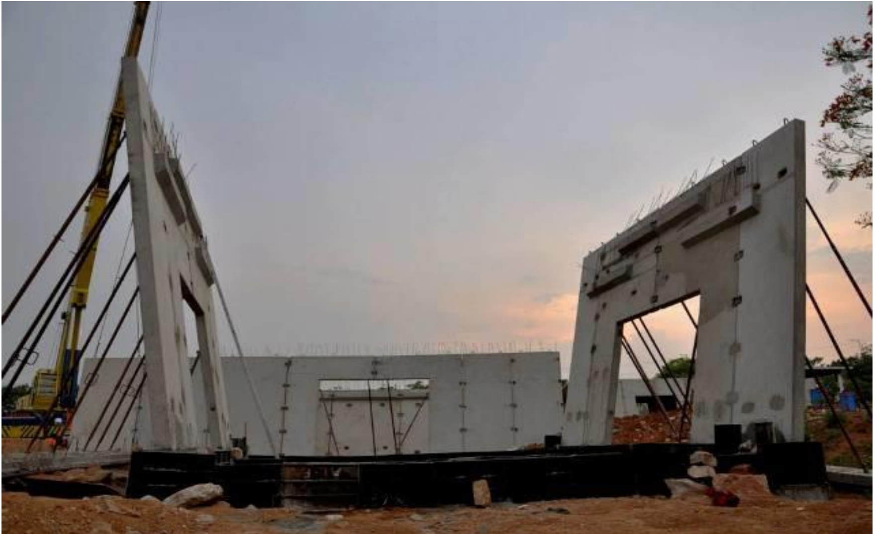
Erection works in progress
