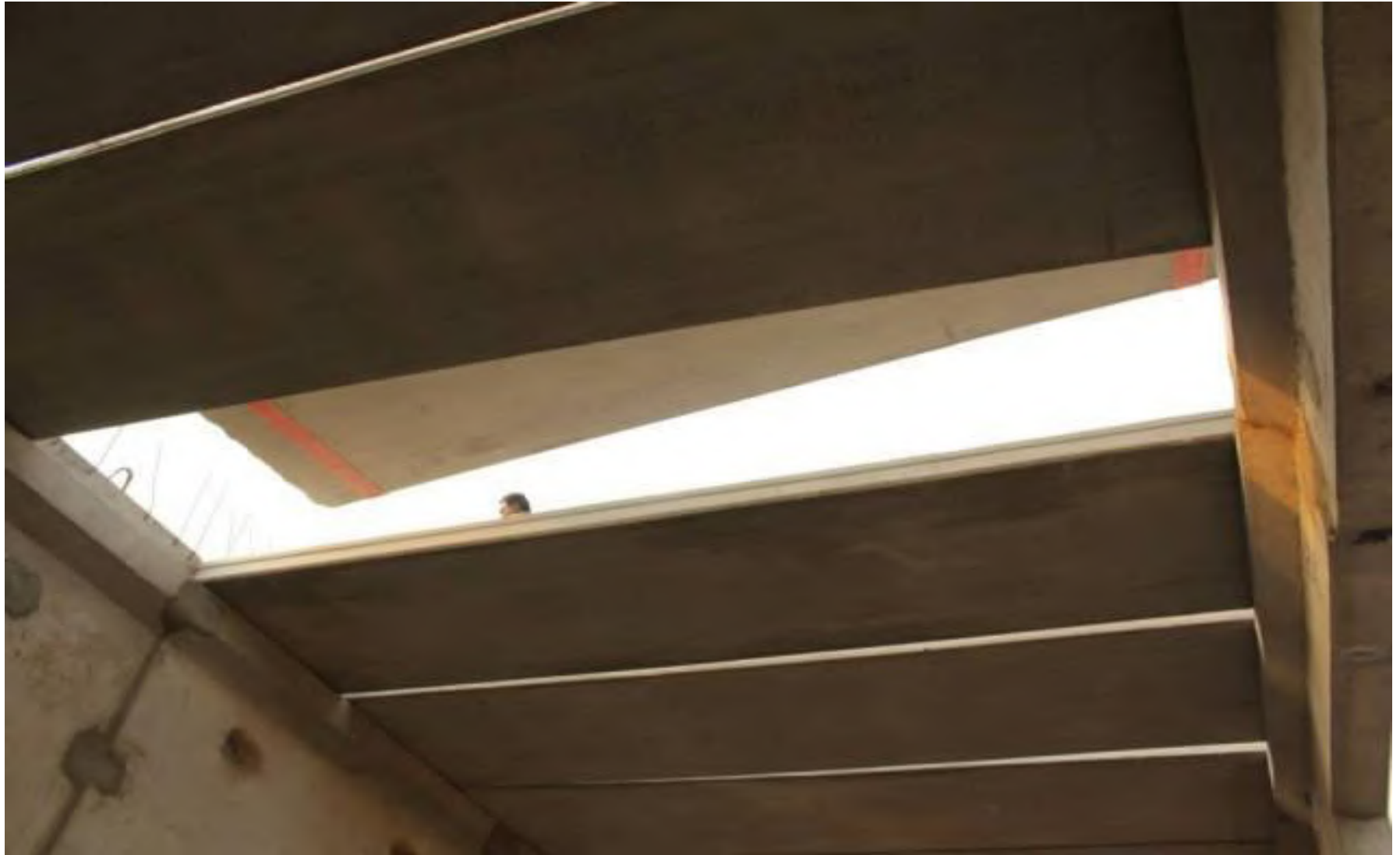
Erection works in progress
